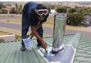
You can then apply Megabond waterproofing over your flashing and roof tiles.
