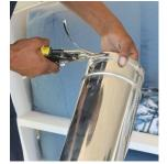
Measure the flue, to make sure, and cut off any excess flue, if needed.
