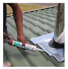
Silicone the edges of the aluminum flashing as well as where the rubber and flue meet.
