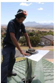
\* Slide the EPDM waterproofing over the insulated flue and connect your cowl on top of the flue.
