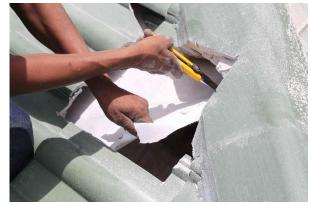
Remove the appropriate roof tiles to make a clear pathway for the chimney/flue.
