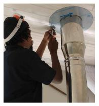
Slide the ceiling plate up along the single flue, onto the double, and then secure it to the ceiling.
