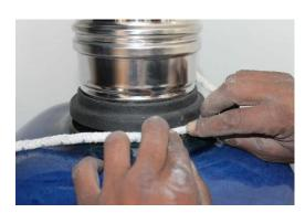
\* If in the case of an Earthfire Firepot, insert the fire rope at the base of the flue before leveling.
