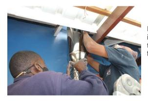
Place the ceiling plate in position and place the insulated flue through the ceiling plate and through the roof. Connect the insulated flue and the normal flue.
