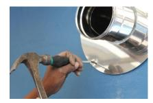
You can attach the outside ceiling plate to the wall, using screw, wall plugs and silicone.
