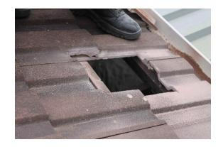
Using the guide hole, cut a square and remove the appropriate roof tiles to make a clear pathway for the chimney/flue.
