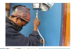
Add PVC pipe brackets to secure the pipe to the wall. Make sure the tap stays open.
