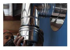
Connect the condense collector to the bottom part of the t-piece, then connect flexible PVC pipe to the condense collector tap.
