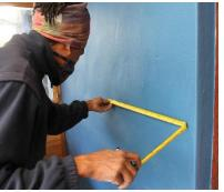
Make sure to measure both sides of the wall to make sure that no beams or any other obstructions are in the pathway of the flue. If there are, you will need to relocate the fireplace or use bends to offset the flue. If not, then you're good to go.
