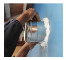
Wrap the insulation blanket around the flue that is in your wall and make sure the flue pipe is level.
