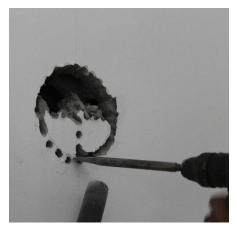
Using a Brutal Hammer Drill, go along the, already drilled, holes to remove the wall.
