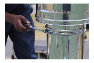
Connect any other insulated flue if needed, then connect the cowl to the insulated flue by using clamps. Make sure the cowl is tight and secured to the flue.
